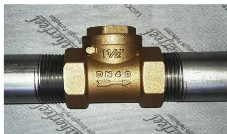
valve is attached. The valve does not let the water flow in both directions and keeps the water trapped in the aqua silencer.
